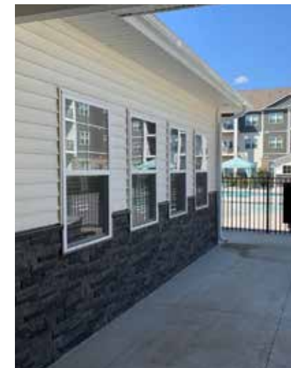
Stacked Stone - Lewiston Crest
