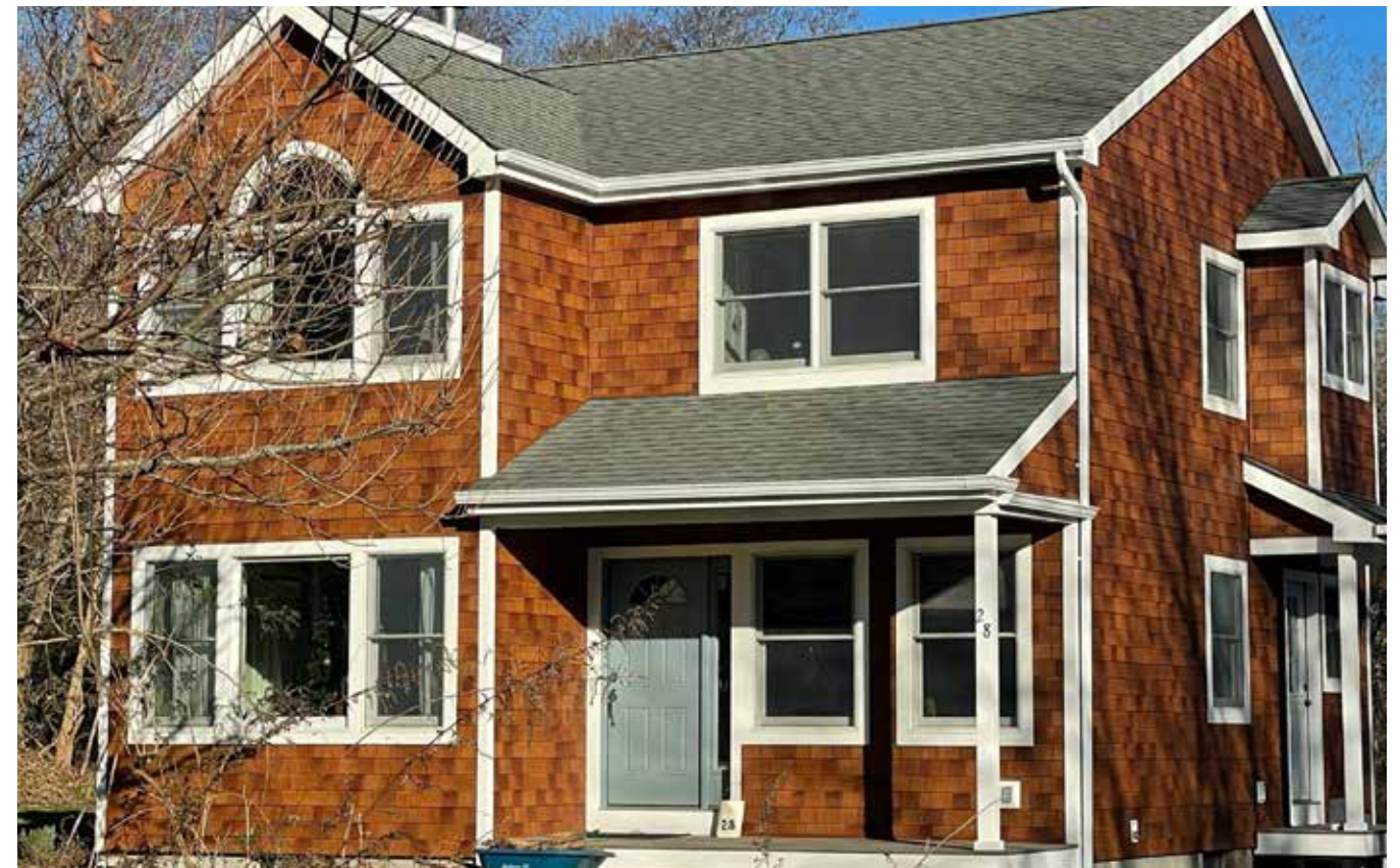
AFTER With Beach House Shake Pacifica Installed
